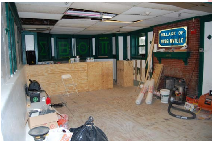
The basement in the middle of construction.
